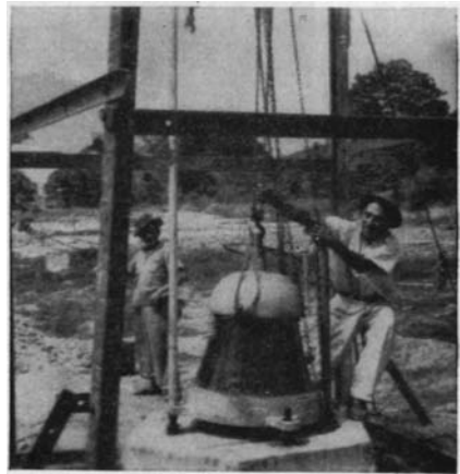
FIG. 2.62. The first step in the construction of a guyed vertical radiator for broadcasting—setting the base insulator. This photograph was taken in Peru. (Photograph courtesy of R. E. Lee.)
