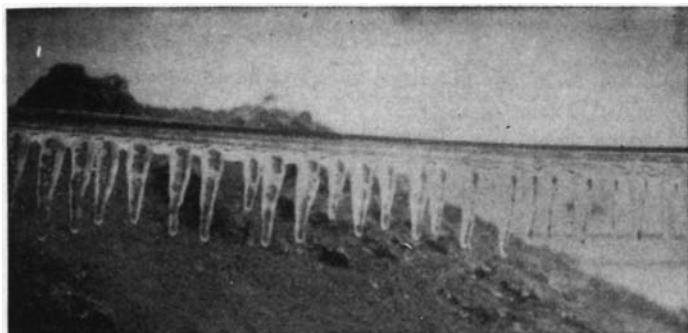
FIG. 1.42. Example of heavy icing on an antenna wire. ( Photograph courtesy of J. S. Hall and C. I. Soucy. )
