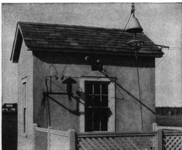
FIG. 1.36. Antenna down-lead and coupling-house-entrance detail as used at medium-power low-frequency stations.
