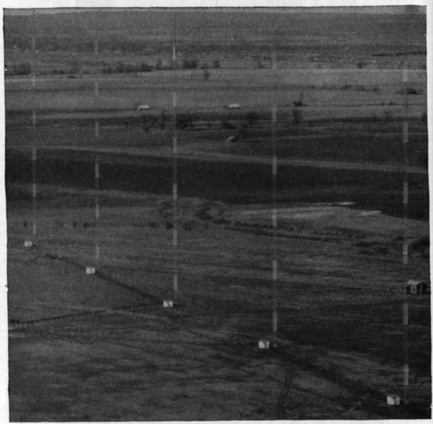
FIG. 2.66. View of Station KTBS six-element directive array. Note pylon antenna for frequency modulation on top of third radiator from the left. ( Photograph courtesy of W. M. Witty, Dallas, Texas. )
