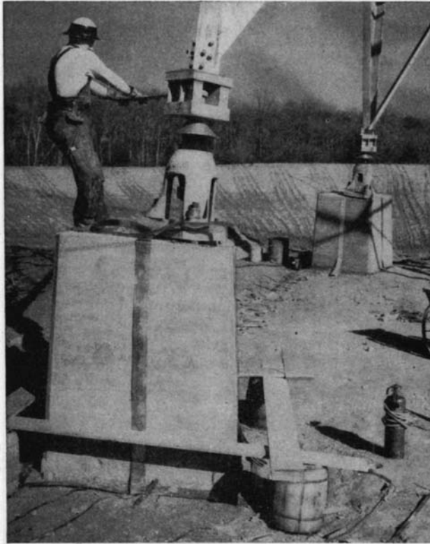
FIG. 2.56. Base of a self-supporting broadcast radiator during construction. Notice tractor and plow tracks in background where ground wires have been plowed into the soil. ( Photograph courtesy of National Broadcasting Company. )
